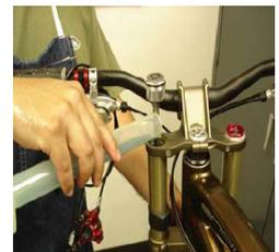
9. Using a 30mm wrench, tighten the cartridge heads into the fork stanchions 87 in-lbs, 9.8 N\*m.
